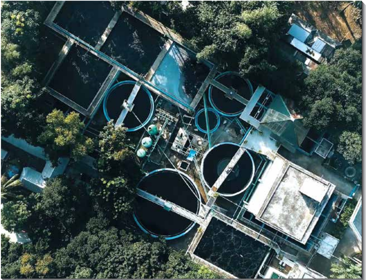
ETP Plant for Safe Environment
